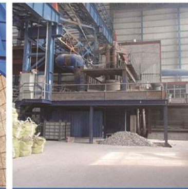
120吨精炼炉 120 tons Refining furnace
